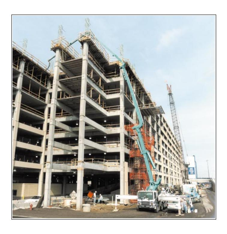
Be the leader in your town with the S 47 SX from Schwing America. With a horizontal reach of 141 feet and a vertical reach of 154 feet, the S 47 SX was designed with operators and owners in mind. The S 47 SX features Schwing's expanded Super-X stabilizers, the industry's first telescoping curved front outriggers. These outriggers telescope into the chassis for compact storage and overall lower structural height. This allows for an optimal
